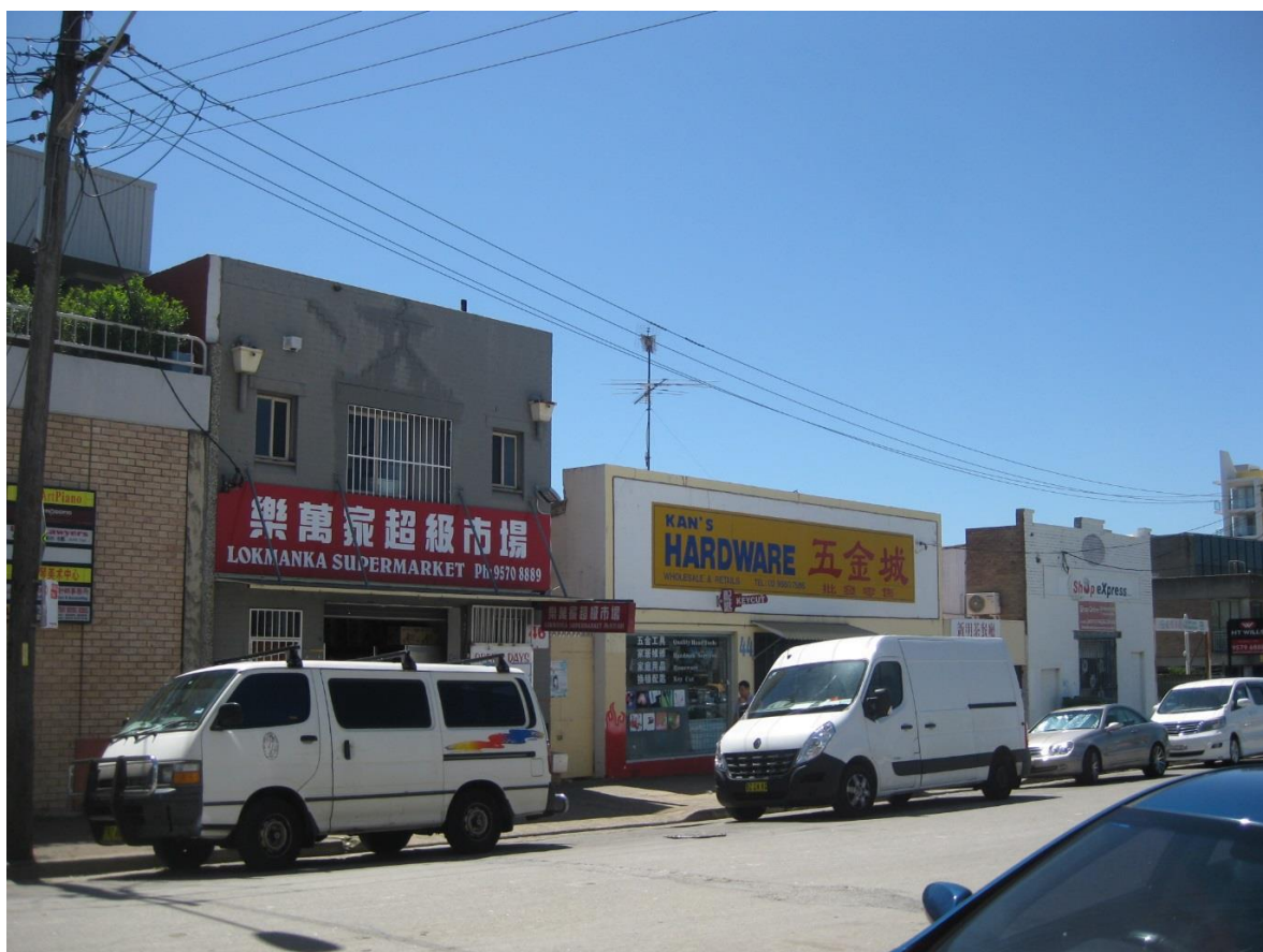
Figure 8: View looking north to one and two storey commercial premises (Source: Google Maps)
